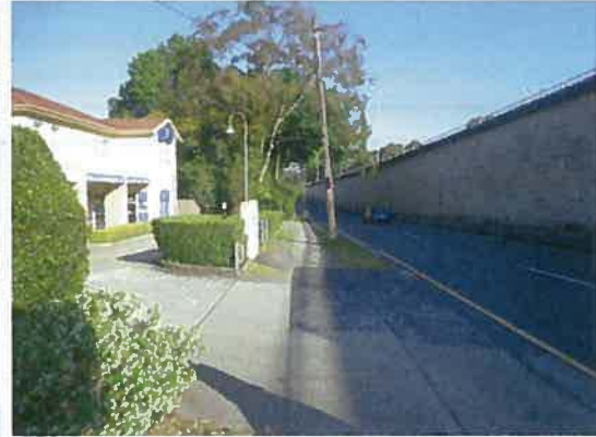
Figure 2.9: Epping Road On-ramp (existing site access)
